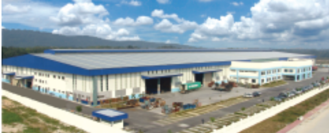
Plant at Kota Damansara Kuala Lumpur
