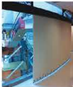
Pathwinder Laterally Sliding Fire Shutter
